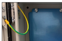
Grounding screw More aesthetically pleasing and safer
